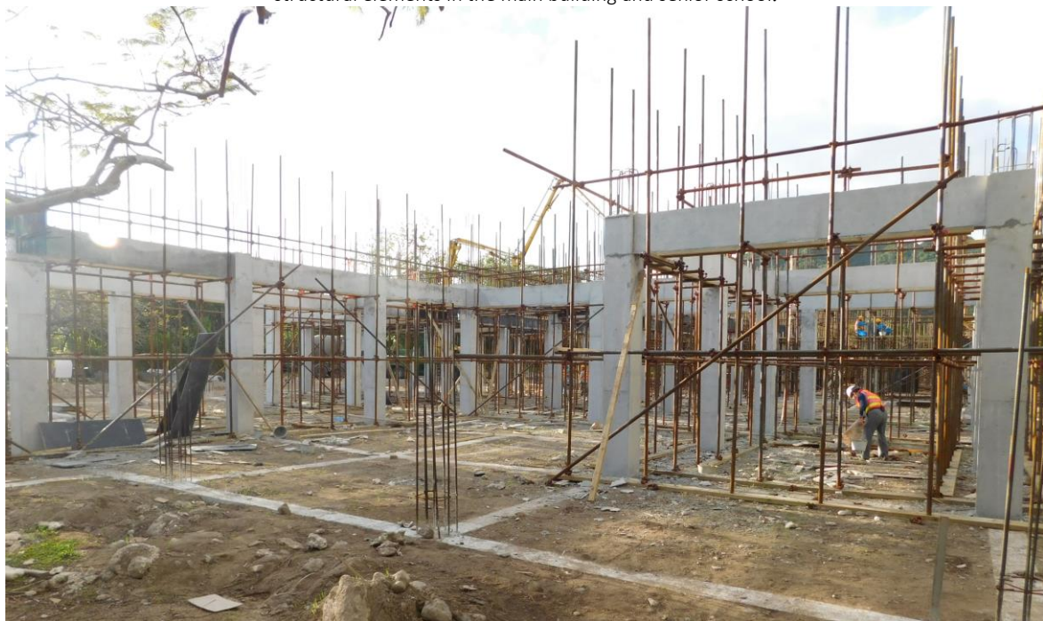
Construction of the main structural elements in the main building.
