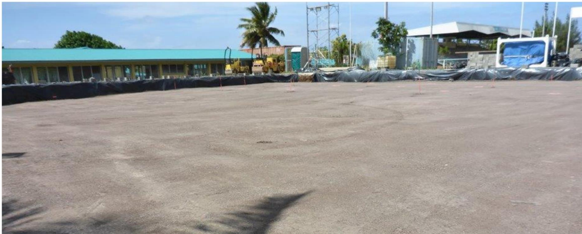
Backfill compaction complete, ready for concrete and steel work.
