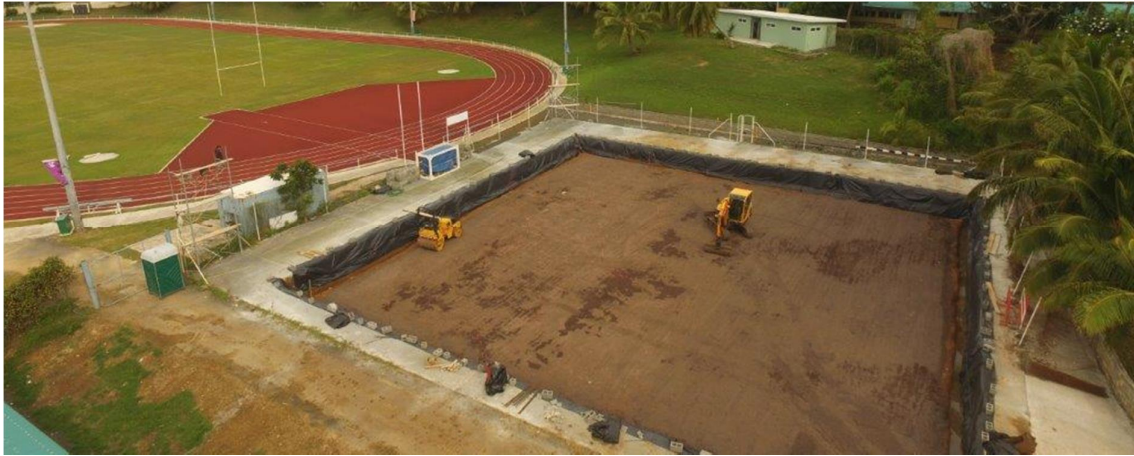
Exposed ground after hard-court and soil excavation.
