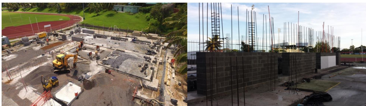
Works on the Technologies Centre progressing well.
