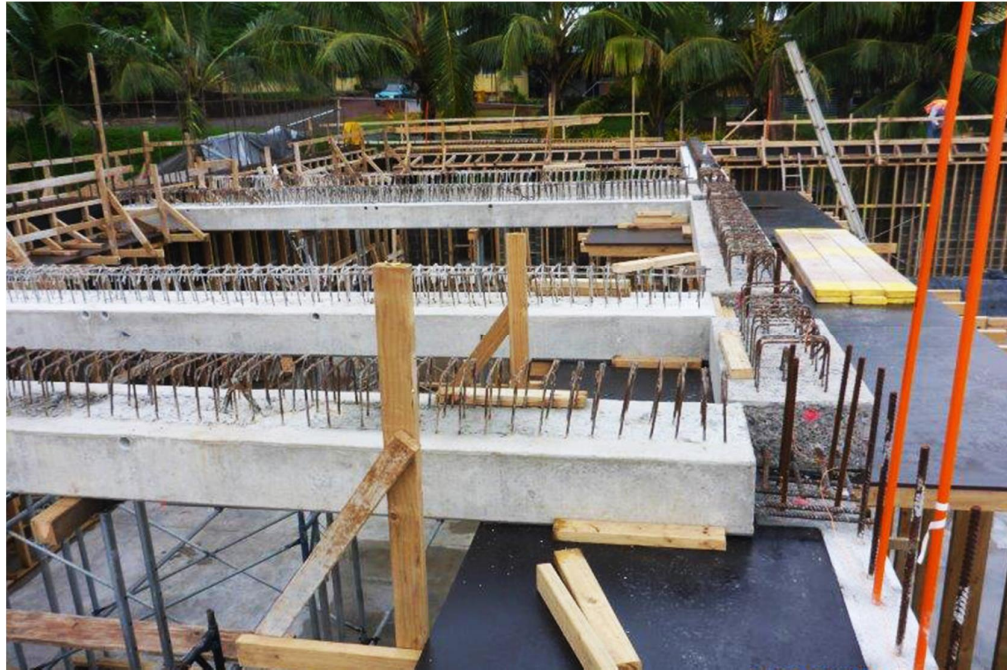
Technologies Centre – Eight beams have been put into place.
